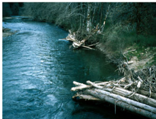
Figure 4. Large wood provides deformable bank protection that allows the channel to absorb the effects of short-term disturbances in the fluvial system and accommodate the long-term impacts of climate or land use change. This figure is available in colour online at wileyonlinelibrary.com/journal/rra
