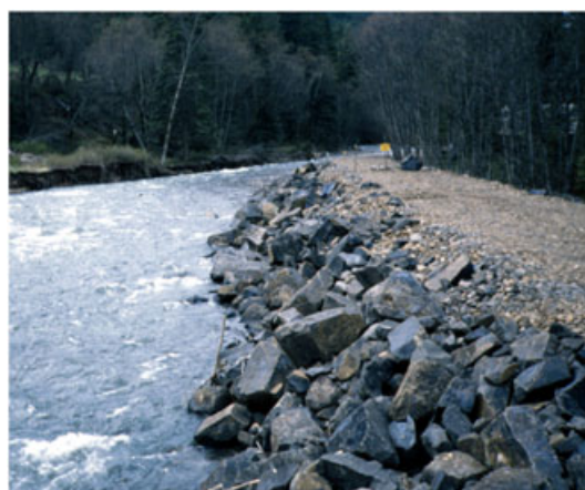
Figure 5. Riprap provides rigid bank protection that reduces the capacity of the channel to absorb the effects of short-term disturbances in the fluvial system and accommodate the impacts of long-term evolution. This figure is available in colour online at wileyonlinelibrary.com/journal/rra
